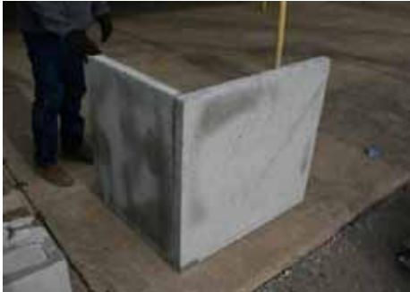
Step 5 - Place end panel and final end bracket.
