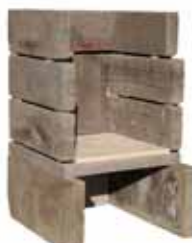
Step 8 - Install floor firebrick
