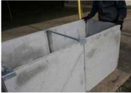
Step 5 - Place end panel and final end bracket.
