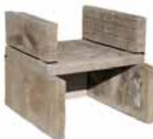
Step 8 - Install floor firebrick
