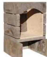
Step 14 - Complete chimney &amp; add hearth
